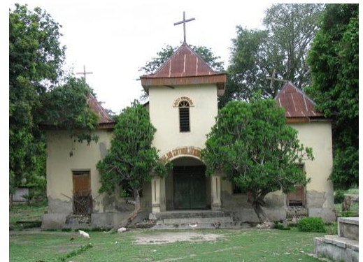
The Church before the earthquake
